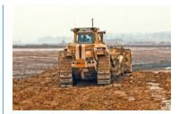
had to be excavated and another three million cubic meters were filled. On this construction site -besides the D11-R-the company uses Topcon 3D GPS+GLONASS levelling systems on:
